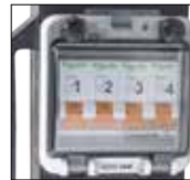
Each output is MCB protected.
